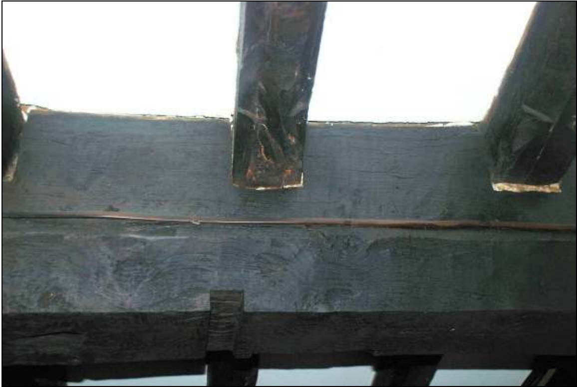
Plate 17: Slot cut in base of ceiling beam, looking west
