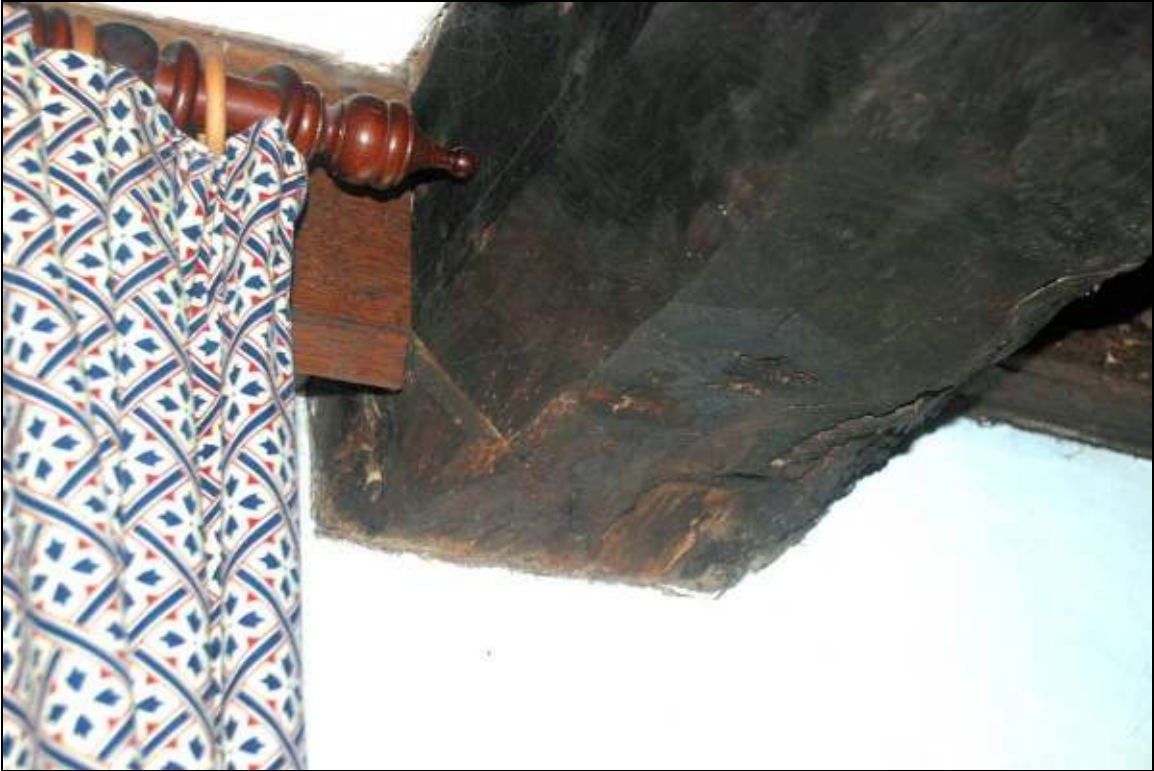
Plate 15: Chamfer and stops on the main ceiling beam looking north
