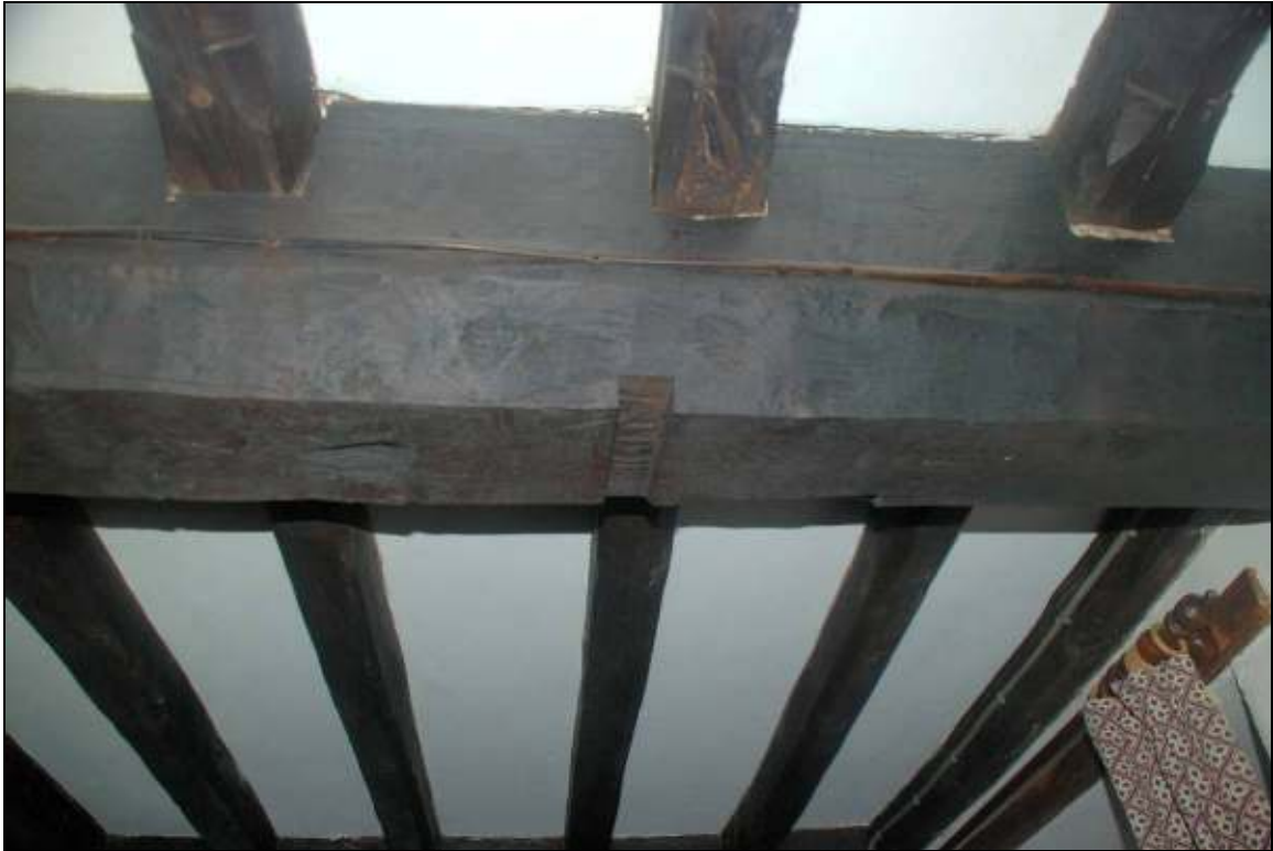
Plate 14: Main room ceiling beam and housed joists, looking west.
