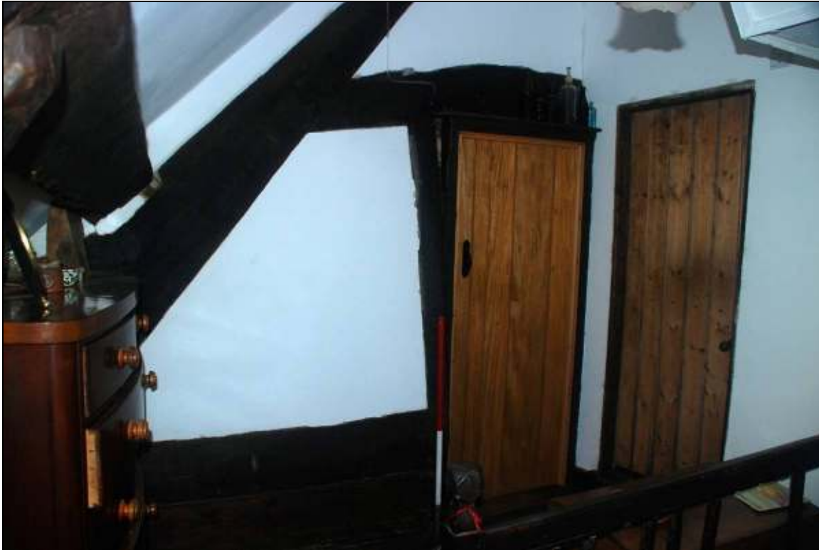
Plate 11: Truss 3 looking west.
