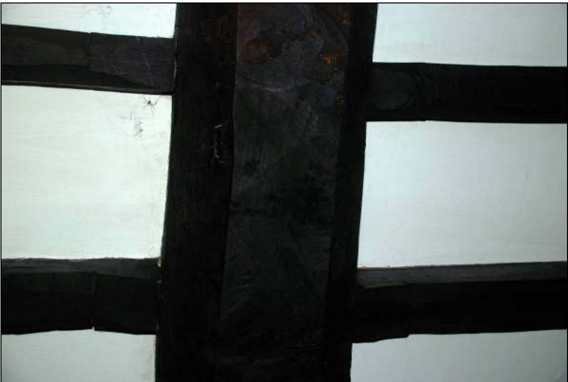
Plate 15: Chamfer and stops on the main ceiling beam looking north
