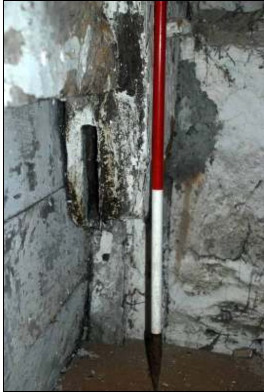
Plate 6: Mortice in foot of northern principal rafter of Truss 1, looking north.
