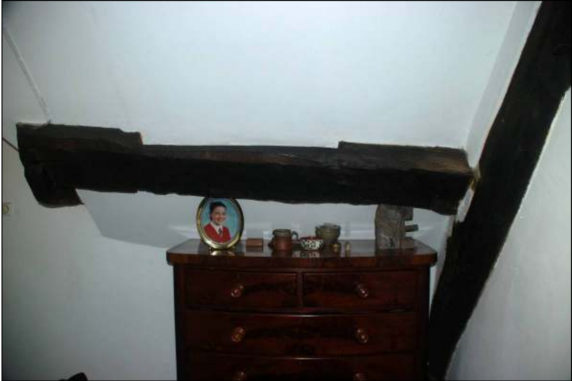
Plate 12: Lower purlin adjacent to Truss 3, looking south.
