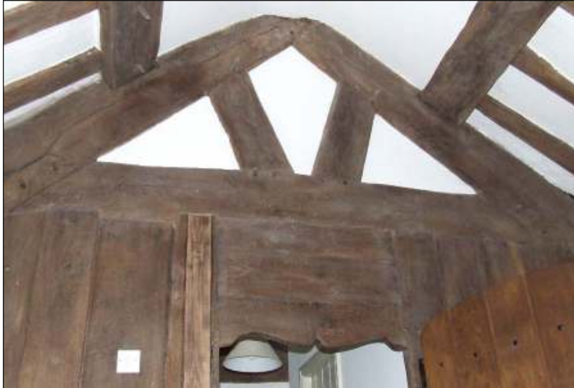
Figure 2: Plank and muntin panel on the first floor, thought to have been moved from the ground floor, with an inserted ogee doorhead.
