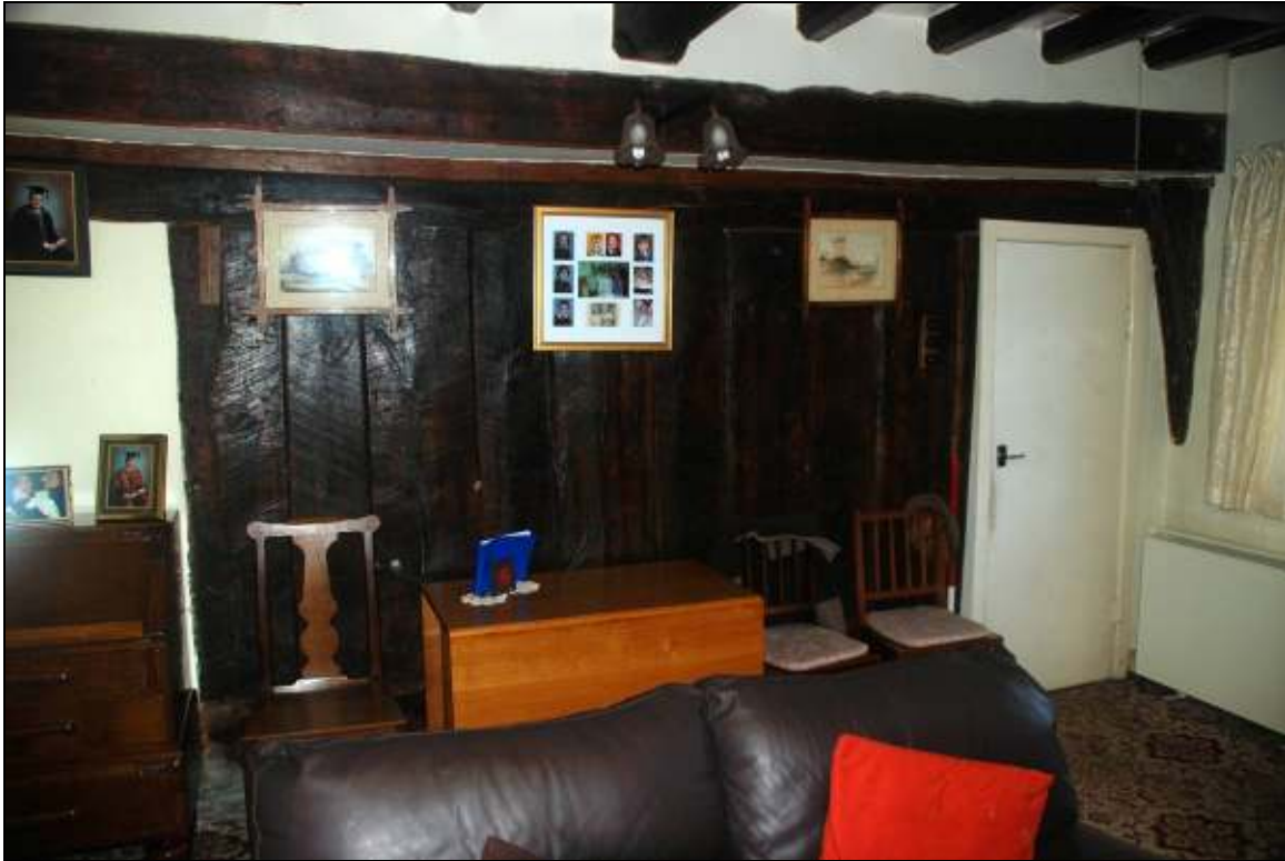
Plate 4: Post and plank partition, looking NNE
