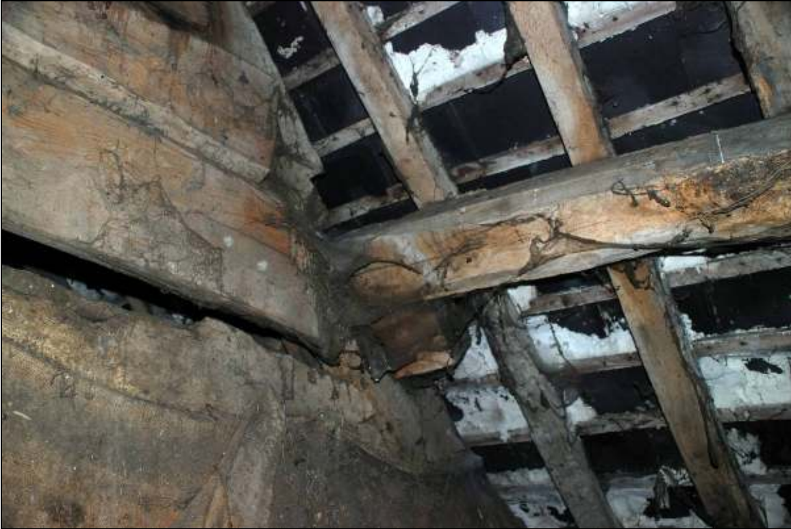
Plate 16: Butt purlins on the barn gable end truss, looking west
