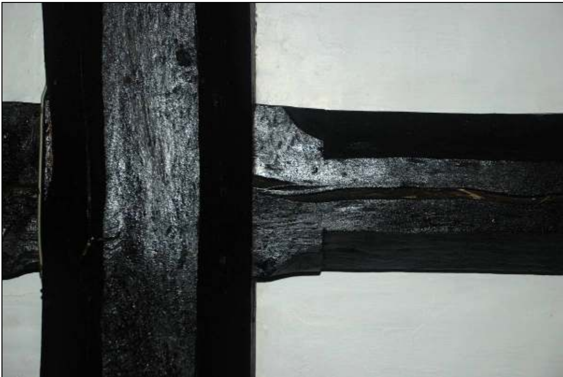
Plate 10: Detail of relationships between the cross beam, and the joists
