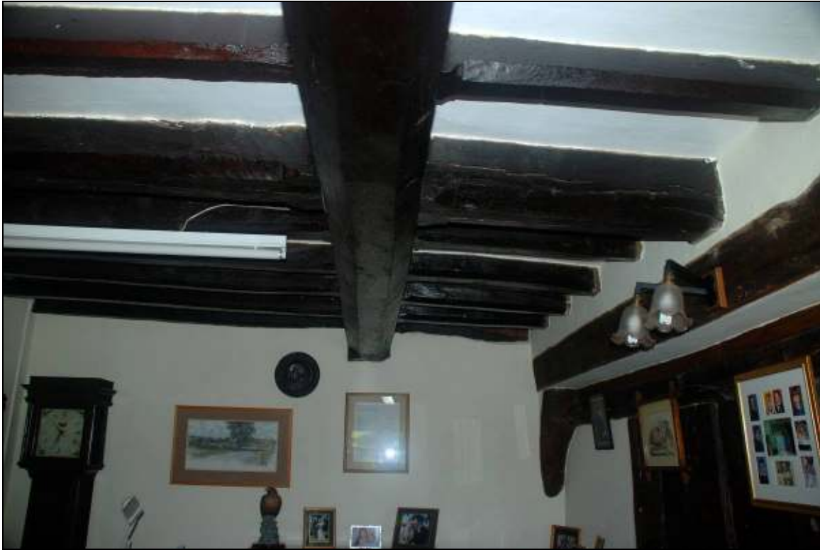
Plate 9: Beamed ceiling in the main ground floor room, looking NW
