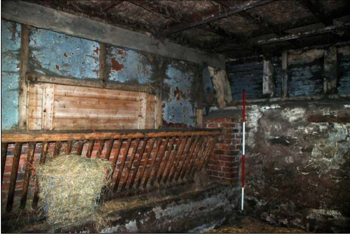
Plate 21: Base of Barn truss 2, looking west
