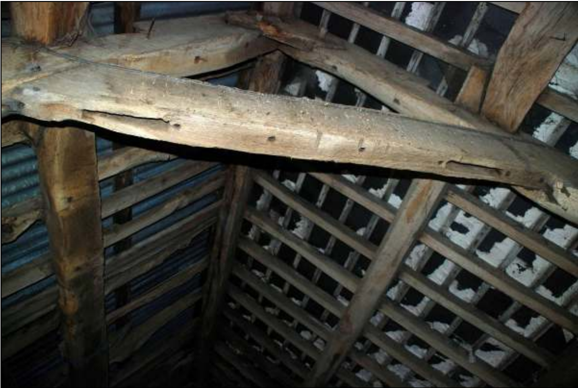
Plate 18: Barn truss 1, possible later tie-beam, looking south
