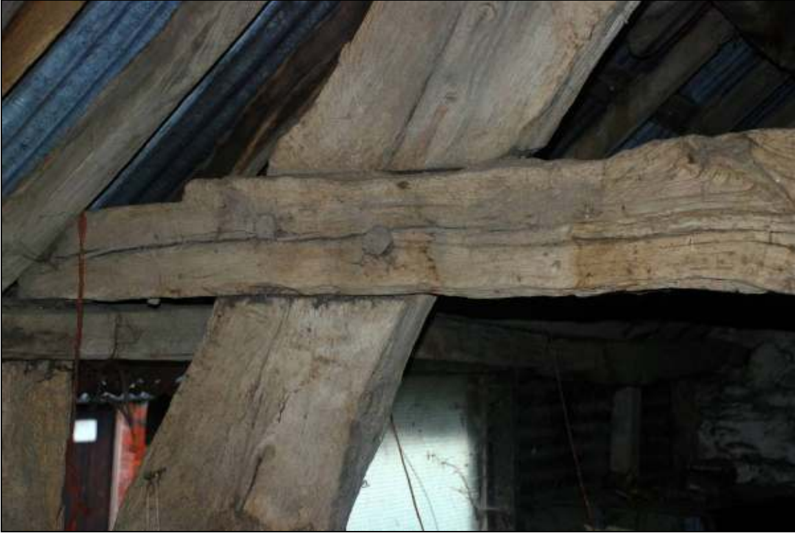
Plate 18: Barn truss 1, possible later tie-beam, looking south
