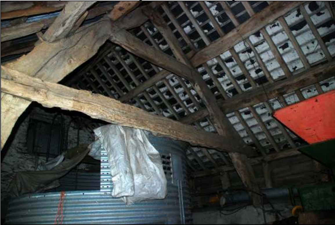
Plate 17: Barn truss 1 looking west
