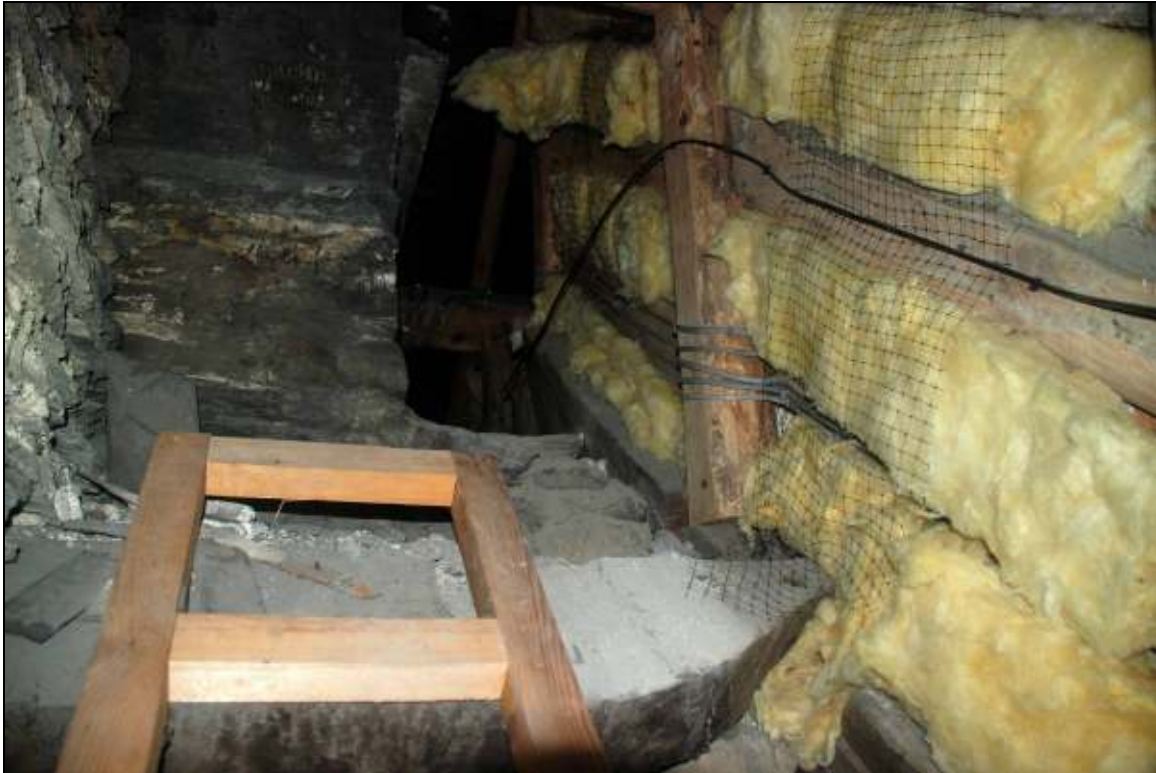
Plate 6: Top of the southern cruck frame, looking NNW and up
