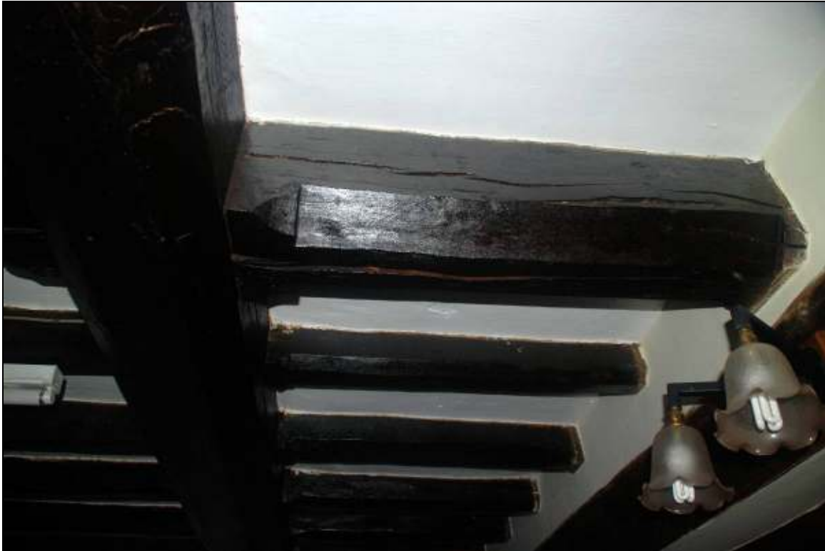
Plate 12: Curved and slightly stepped stops on joists
