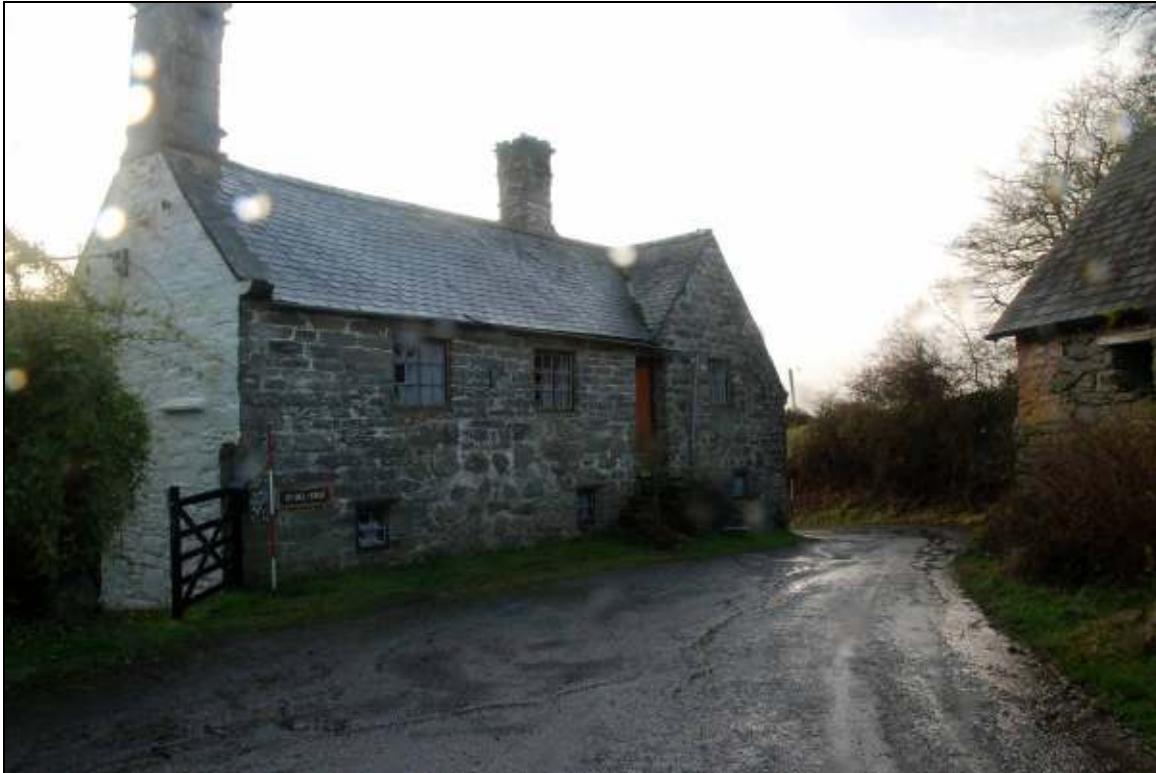
Plate 6: South Wing looking SW
