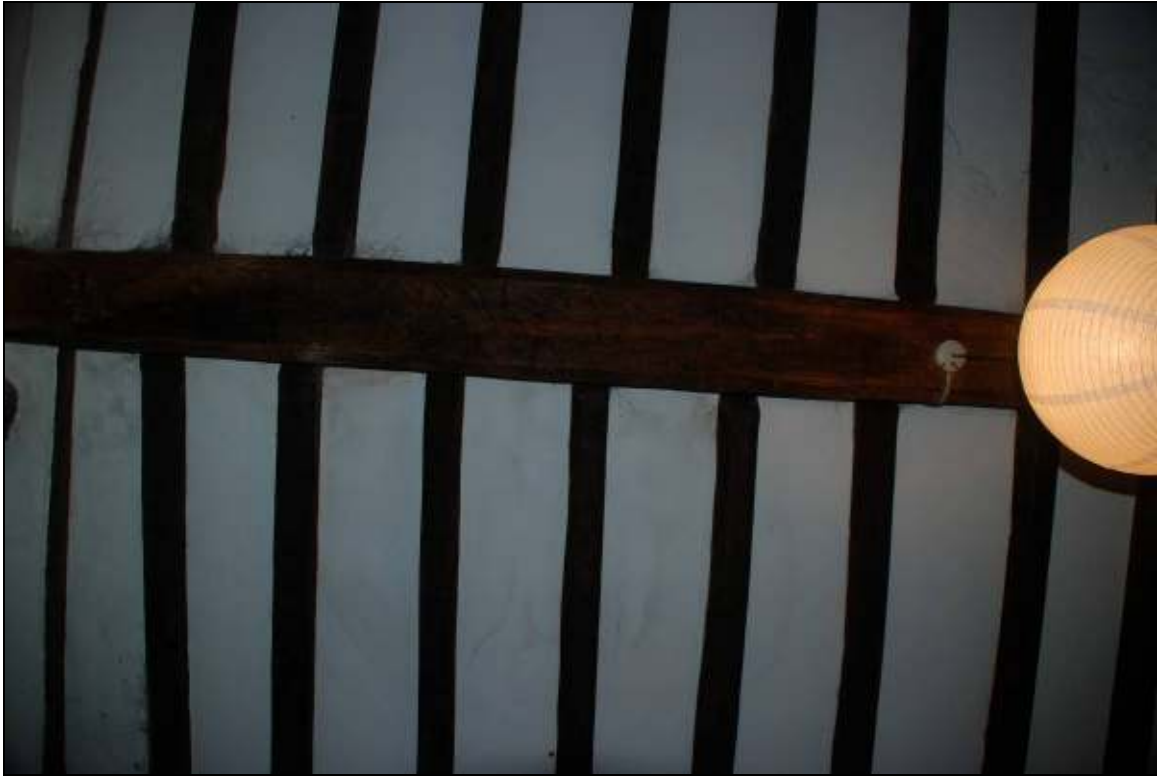
Plate 26: Offset joists in ceiling of southern ground floor room
