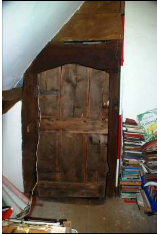
Plate 15: Attic door, looking south
