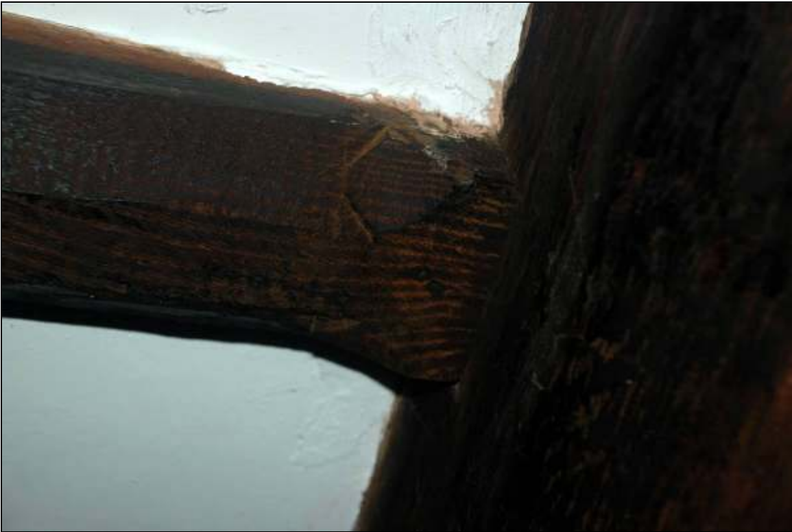
Plate 27: Truncated beam in hallway, looking SW
