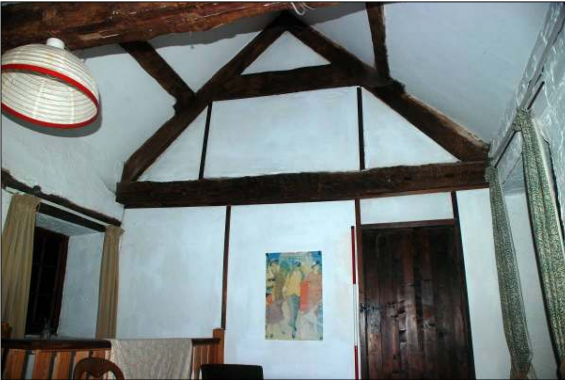
Plate 33: Joint between main beam and coffer in bedroom above the kitchen
