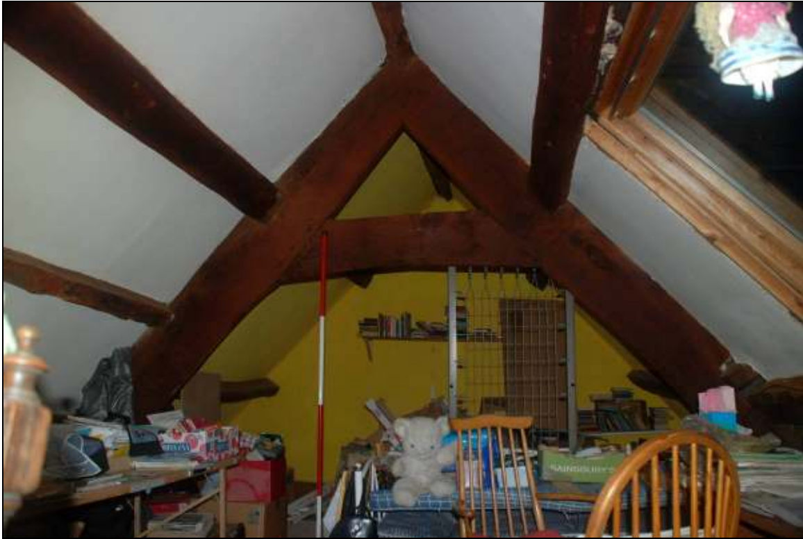
Plate 9: Main range, truss 1, looking north
