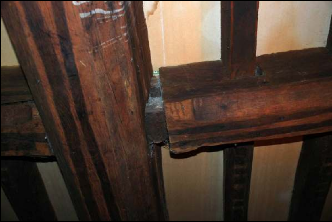
Plate 33: Joint between main beam and coffer in bedroom above the kitchen
