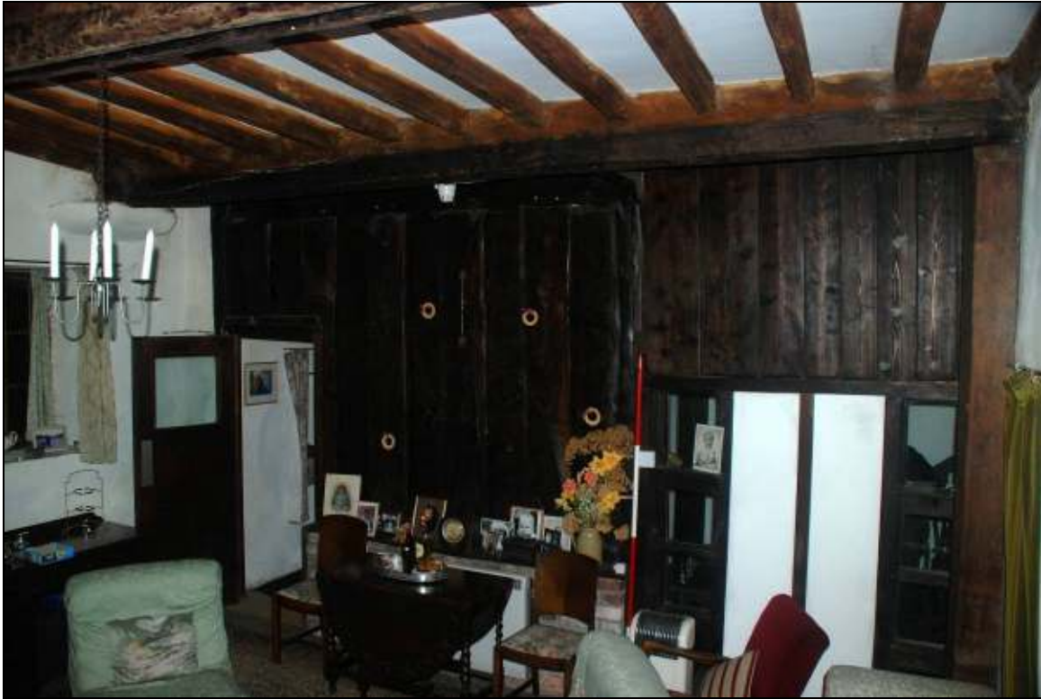
Plate 18: Partition between the main range and the South Wing, looking west
