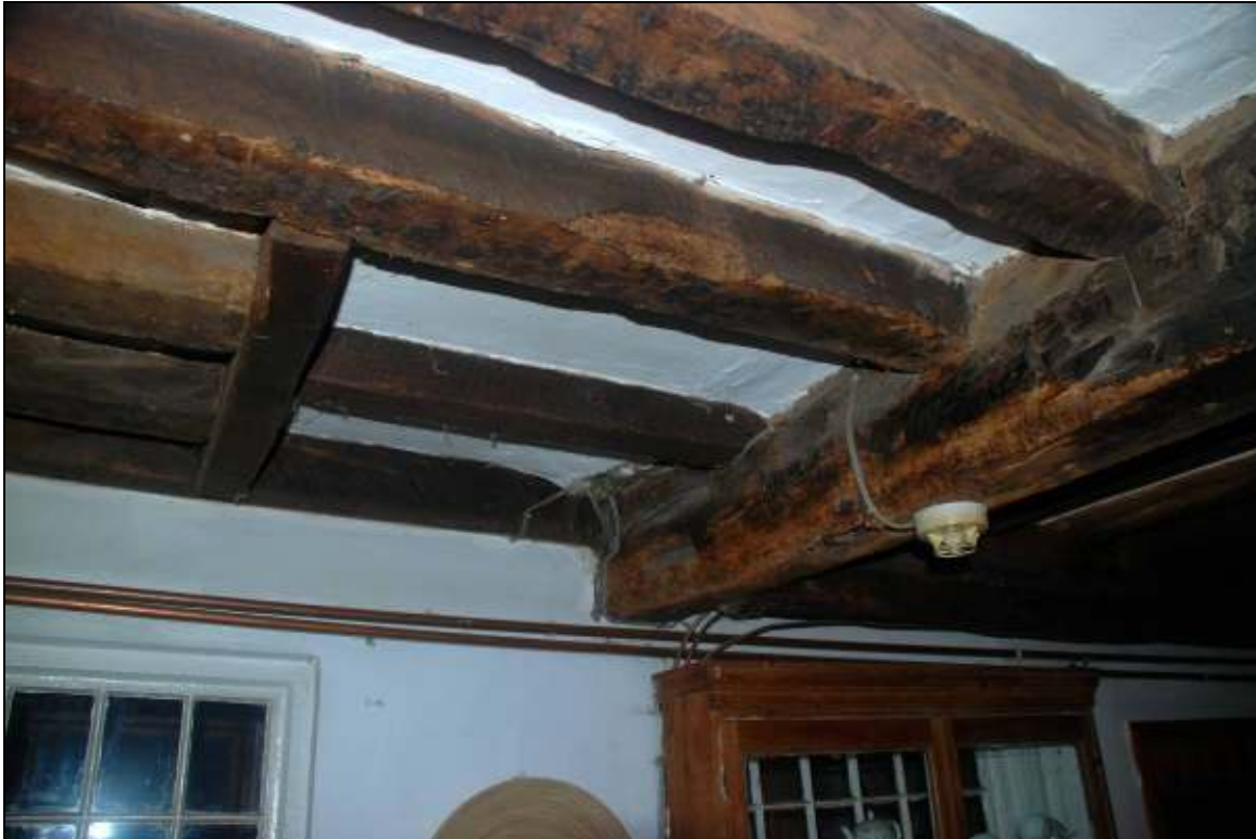
Plate 29: Trimming joist in ceiling of kitchen
