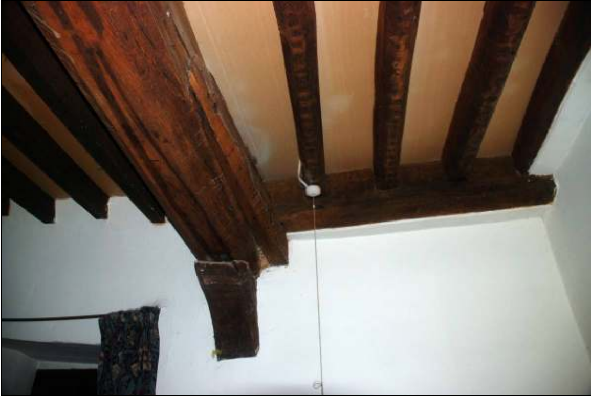
Plate 32: Beam resting on wooden supports in bedroom above kitchen, looking west
