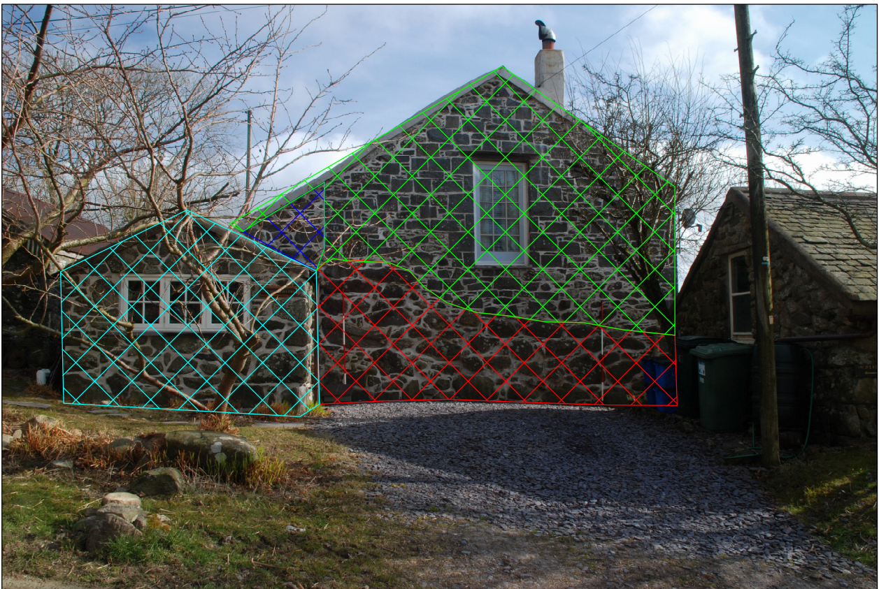
Western gable end
