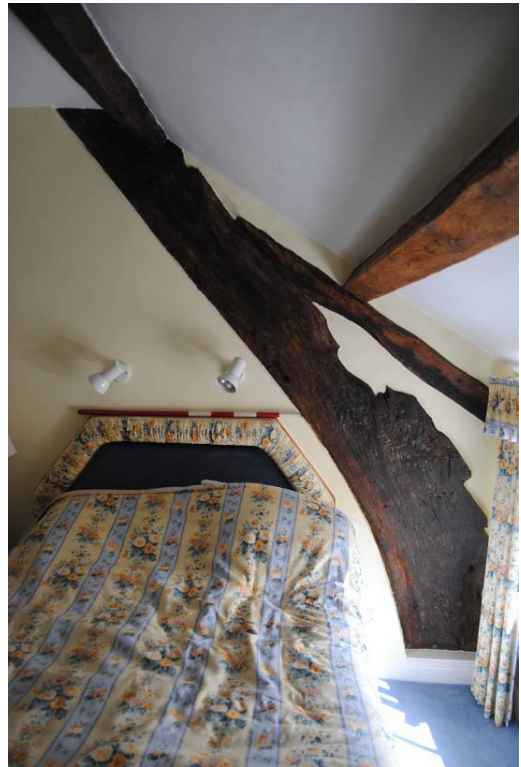
Plate 19: Cruck [T2] (S); Room [1F04] looking east.
