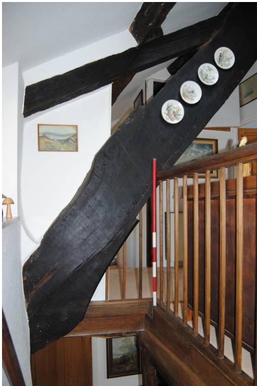
Plate 20: Cruck [T3] (N); stairwell, [deni3] dated to Spring 1488.
