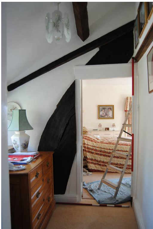
Plate 24: Cruck [T4] (N); [1F01].
