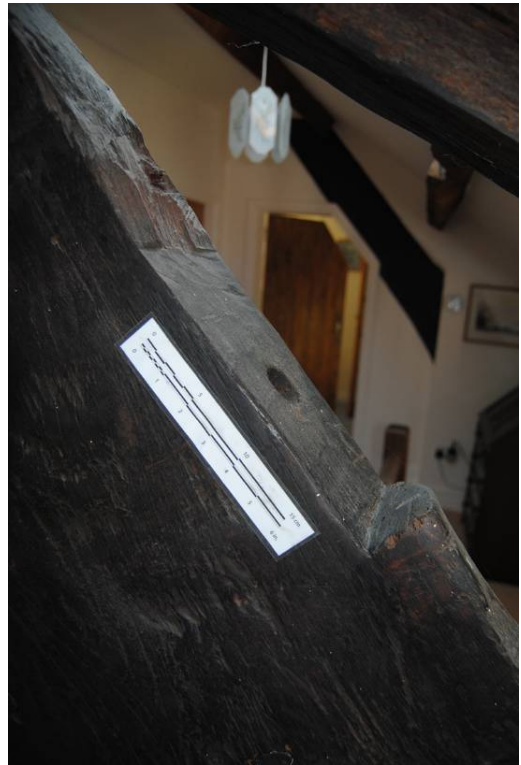
Plate 21: Primary purlin housing at [T3] (N).
