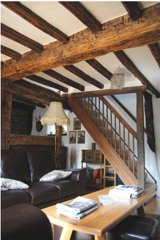
Plate 14: Inserted stair, [GF02].
