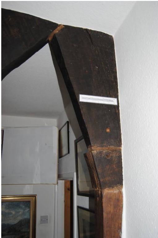
Plate 22: Cruck [T3]; truncated collar and northern V- strut, [1F01].
