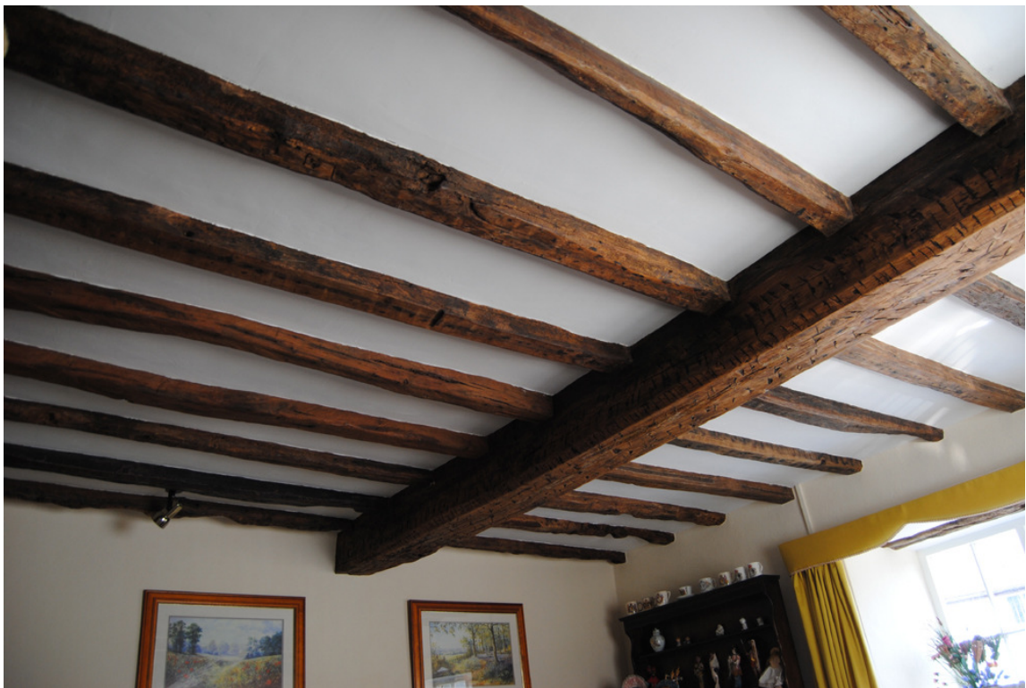
Plate 17: Ceiling structure, room [GF05].
