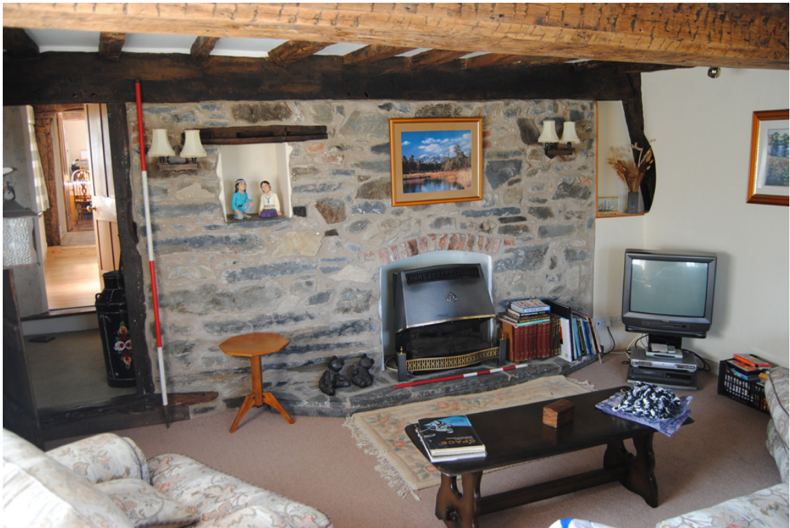
Plate 16: Inserted stack within Room [GF05], looking west.
