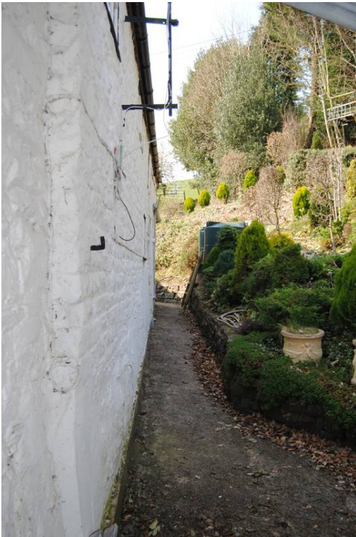
Plate 4: Terracing in of north elevation (1).
