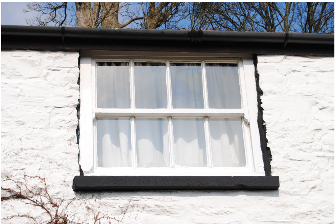
Plate 9: 4/4 horned, double-hung vertical sash.
