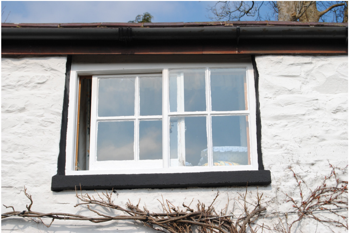
Plate 8: Horizontal sliding sash window.
