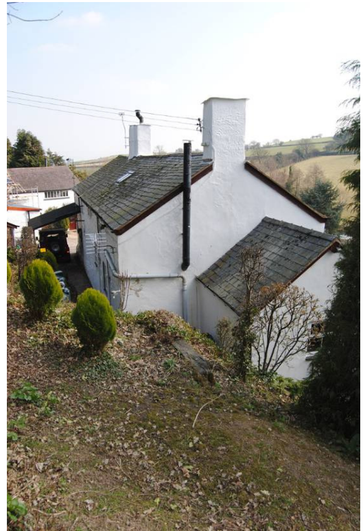
Plate 5: Terracing in of north elevation (2).
