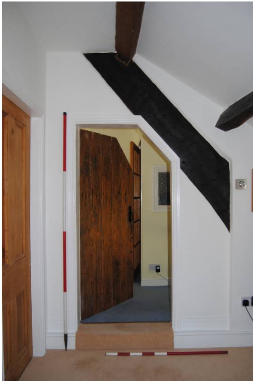
Plate 18: Cruck [T2] (N); Room [1F01] looking west.
