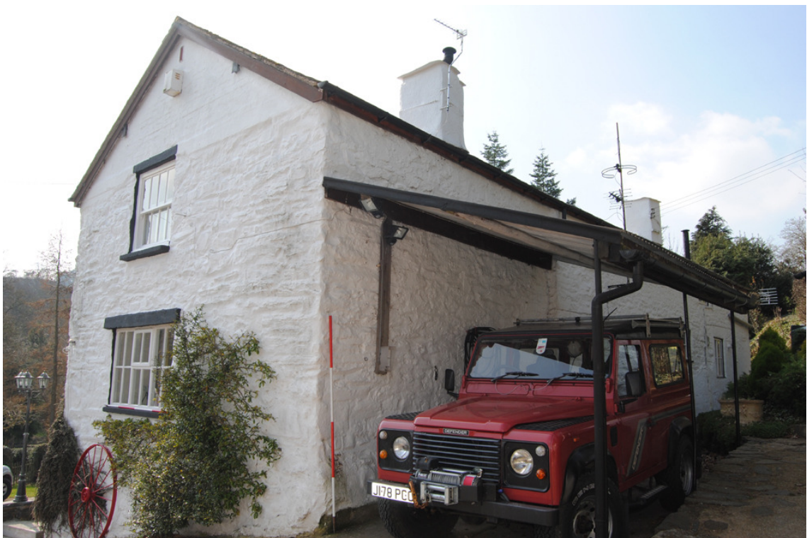
Plate 3: North elevation, oblique, looking south-east.
