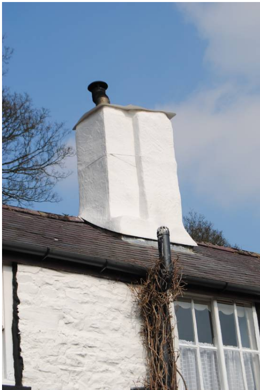
Plate 6: Principal ridge stack.
