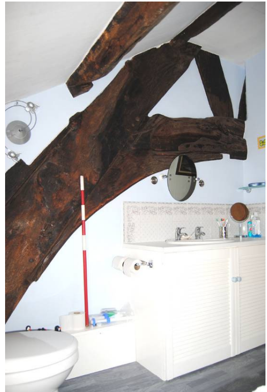
Plate 23: Cruck [T3] (S); surviving collar and arch-brace within Room [1F02]. ([deni4b] dated to winter 1488/89).
