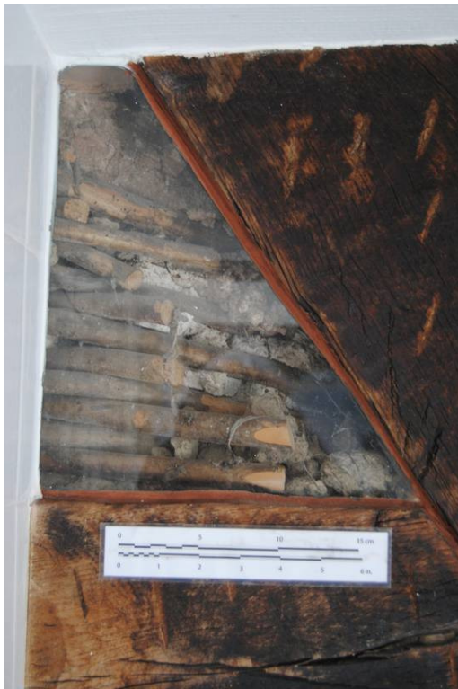
Plate 26: Wattle and daub infill above collar of [T4] [1F02].
