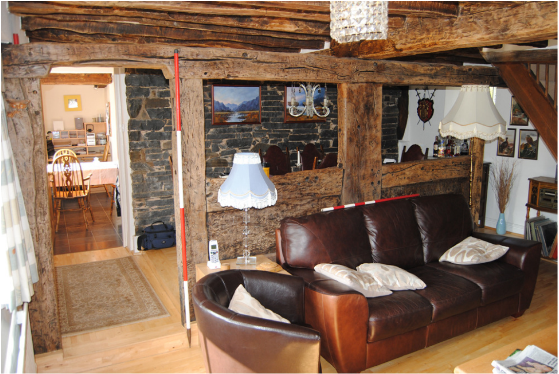
Plate 13: Inserted 'byre' partition within Room [GF02].
