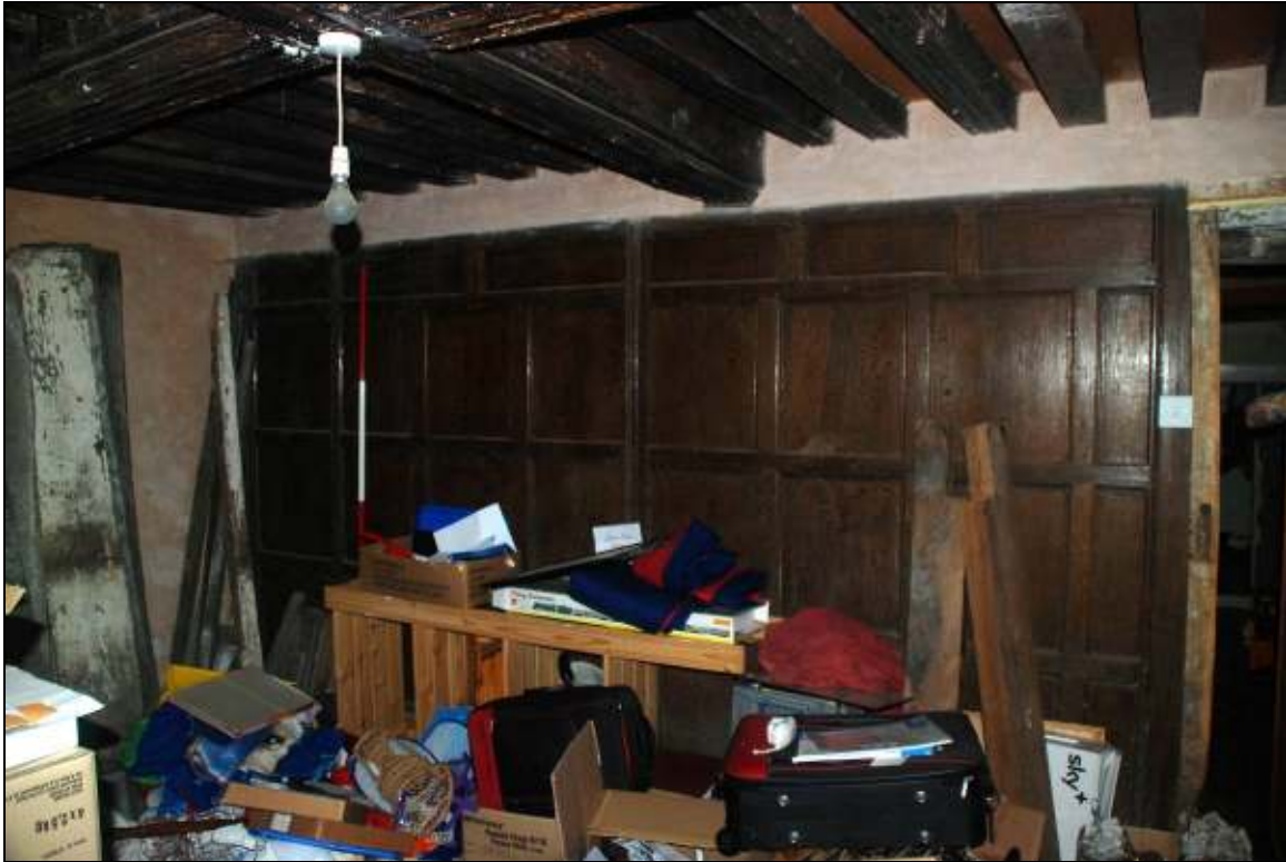
Plate 47: Panelling between the Central and SW ground floor rooms, looking NE
