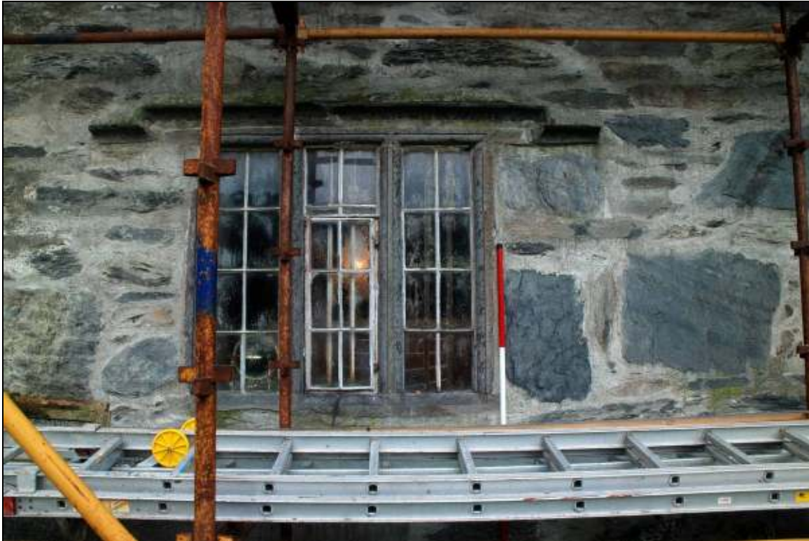
Plate 3: Three light mullioned window, looking NW
