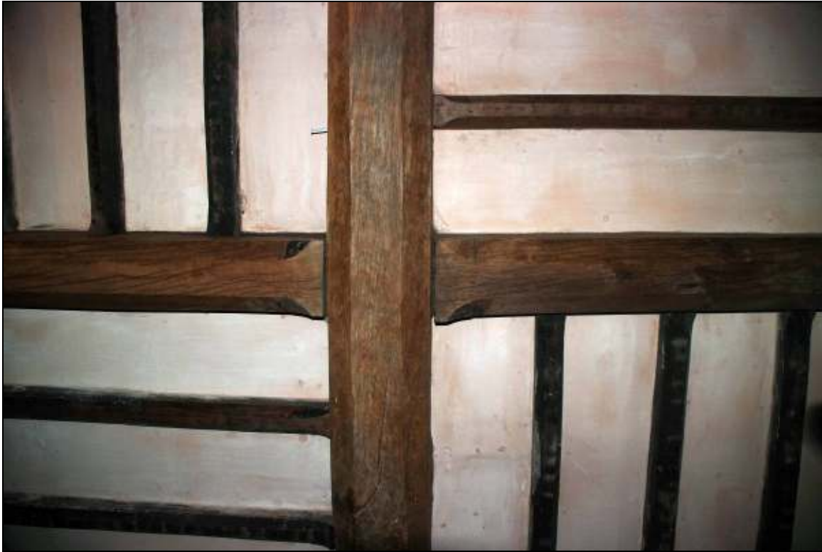
Plate 40: Ceiling of the central ground floor room, looking up
