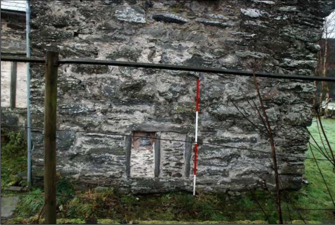
Plate 12: Mullioned window in SW range, looking SE
