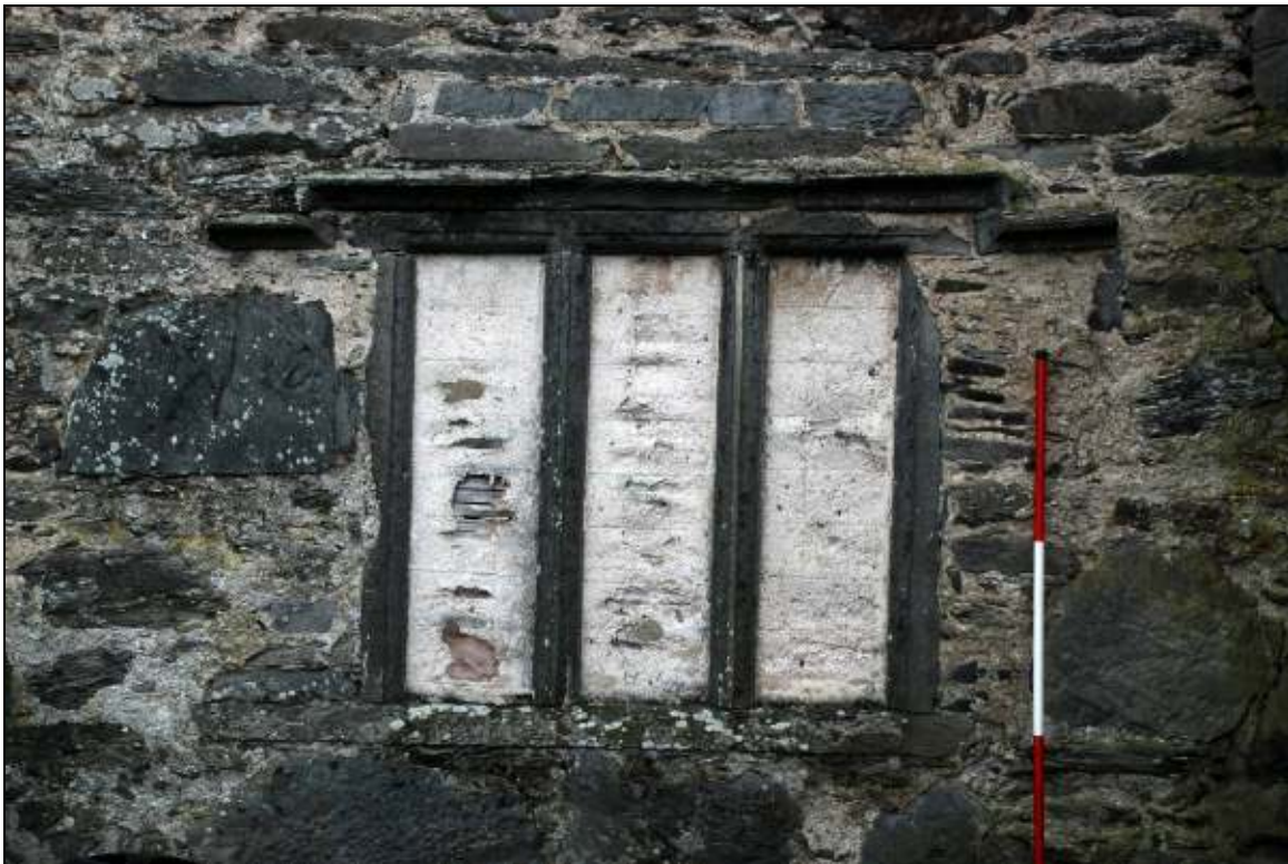
Plate 4: Two light mullioned window, looking NW
