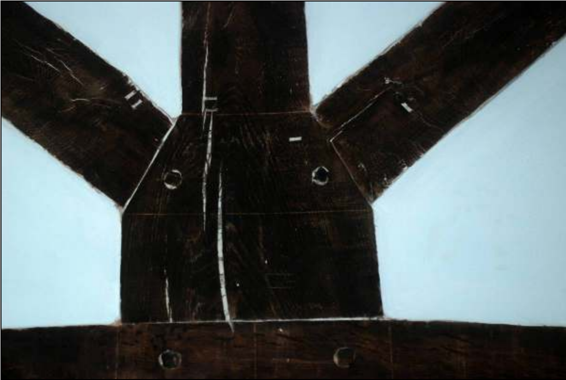
Plate 31: Carpenter's marks on Truss 7, looking NW
