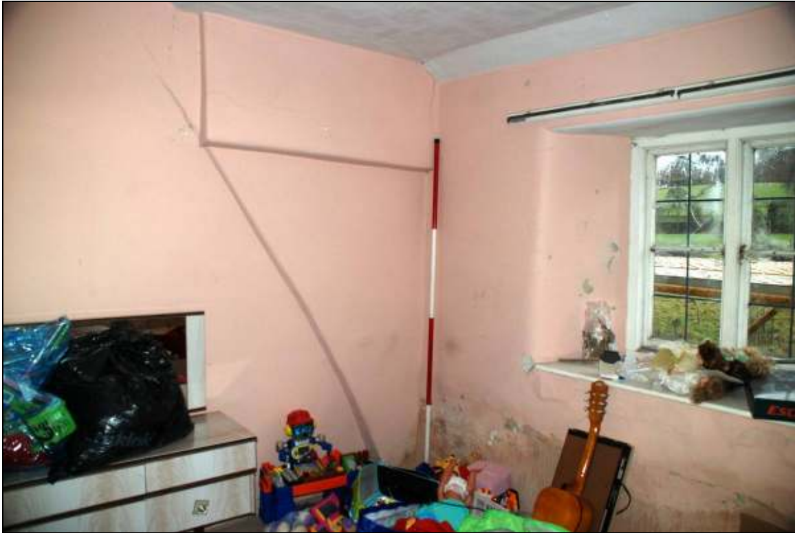
Plate 19: Truss 1, looking east
