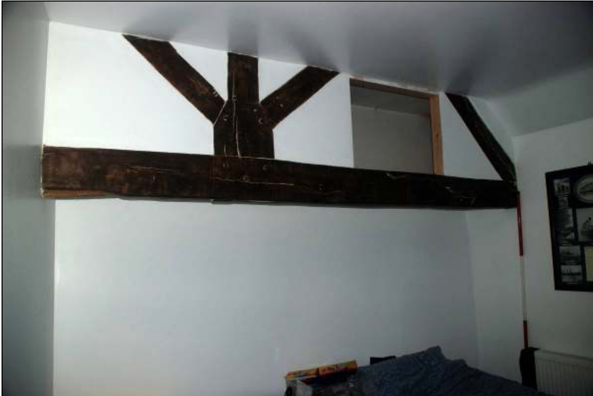
Plate 28: Truss 7 looking north
