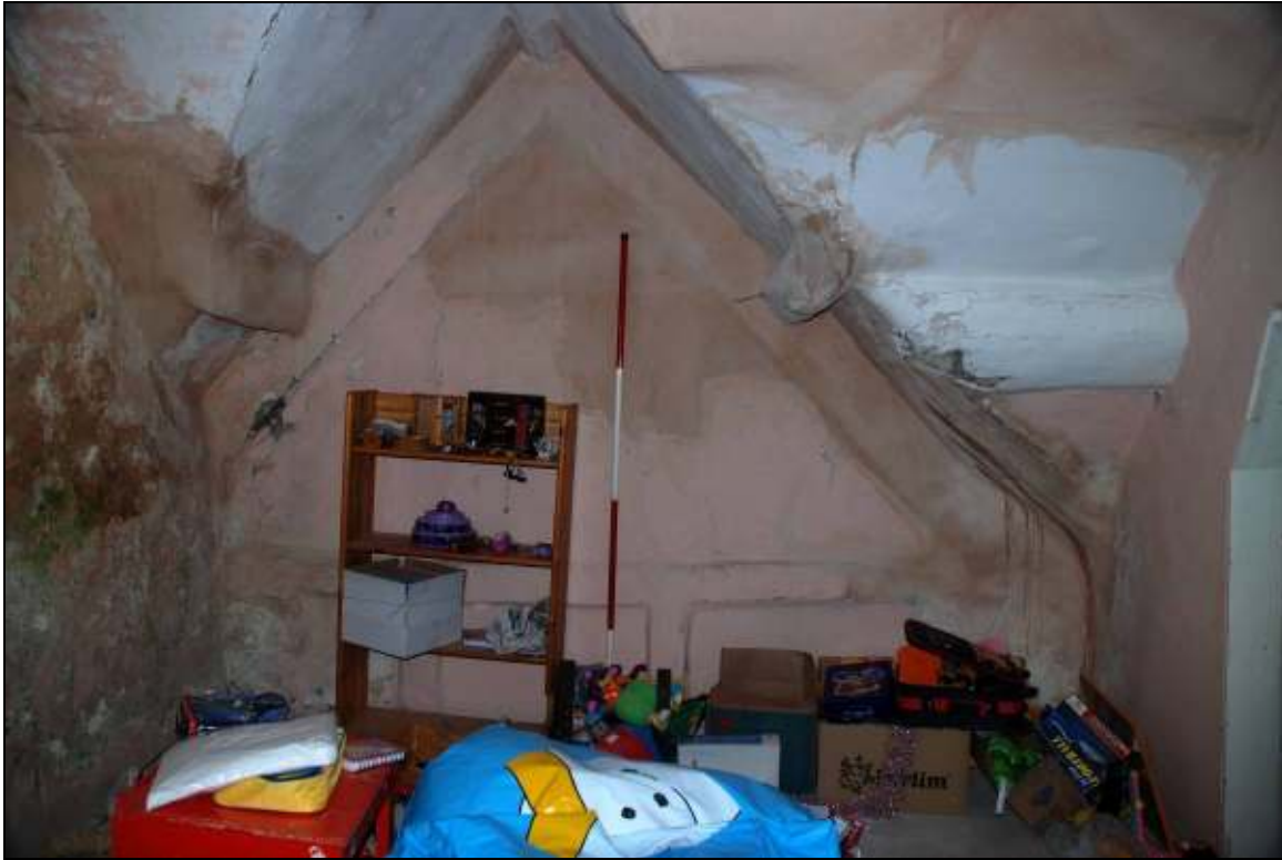
Plate 25: Partition between the main range and the SW Wing, looking NW
