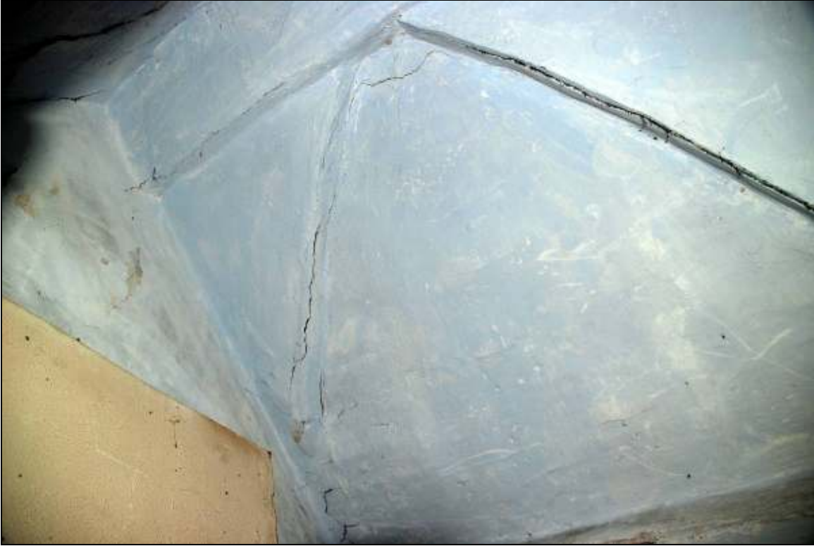
Plate 22: Windbraces below the upper purlin between Trusses 3 and 4, looking west
