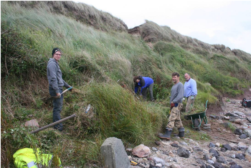
Photo 1: Initial clearance of the sand dunes
