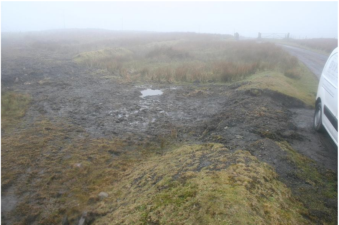
Photo 10: View of damage to the modern bank at the northeast end of the modern trackway across the site. Facing WNW.
