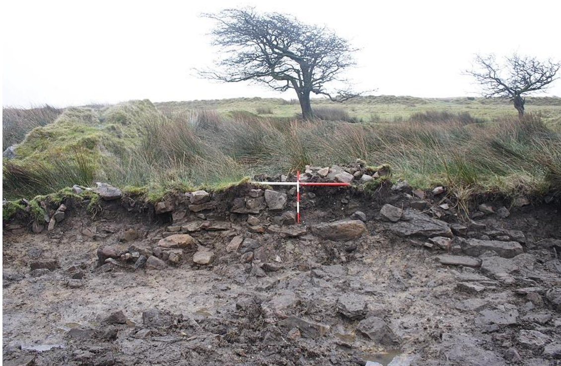
Photo 28: Section showing area of former northeast gable wall and outshot attachment. Facing SE, 1m & 0.5m scale.
