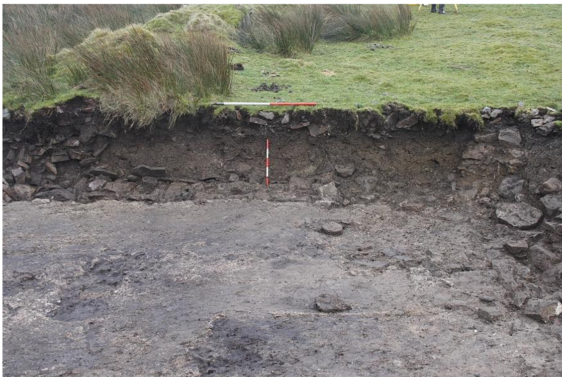
Photo 26: Section at south-western end of the building, showing depths reached by the unauthorised excavation. Facing SE, 1m & 0.5m scale.
