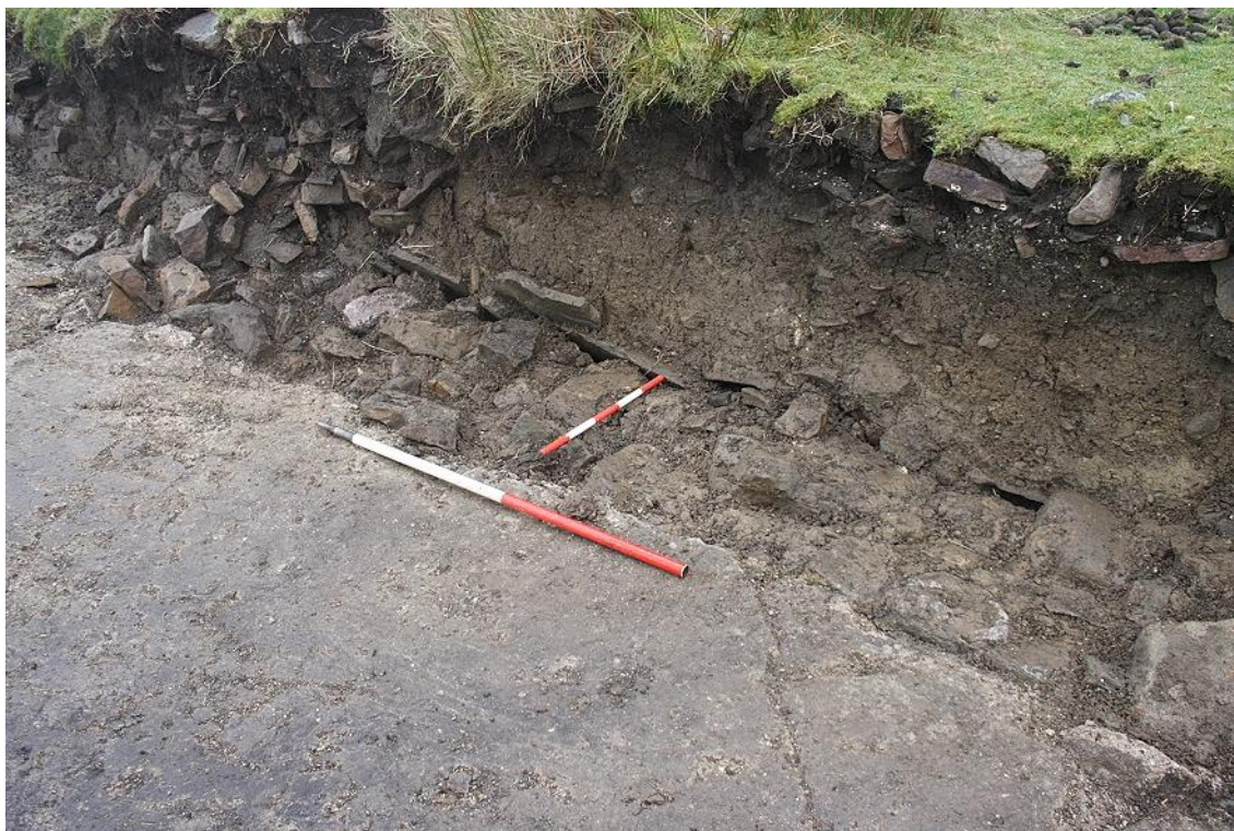
Photo 17: Looking at the north-eastern wall, remains of the stone-flag covering of an external drainage culvert is visible at the base of the section along the outside of the wall. Facing E, 1m & 0.5m scale.
