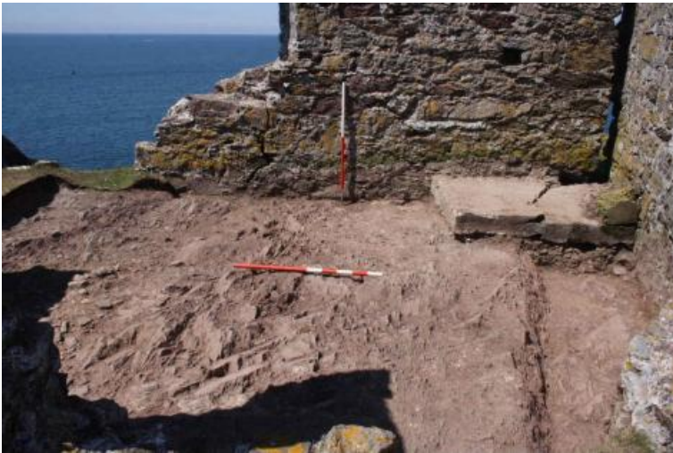
Photograph 7. The interior of the Blockhouse after removal of turf and topsoil showing the concrete plinth in the north-west corner and the foundation trench. Scales 1m.
