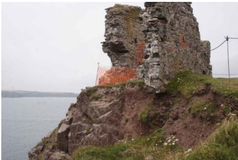
Photograph 3. The undercut east wall at the south end.
