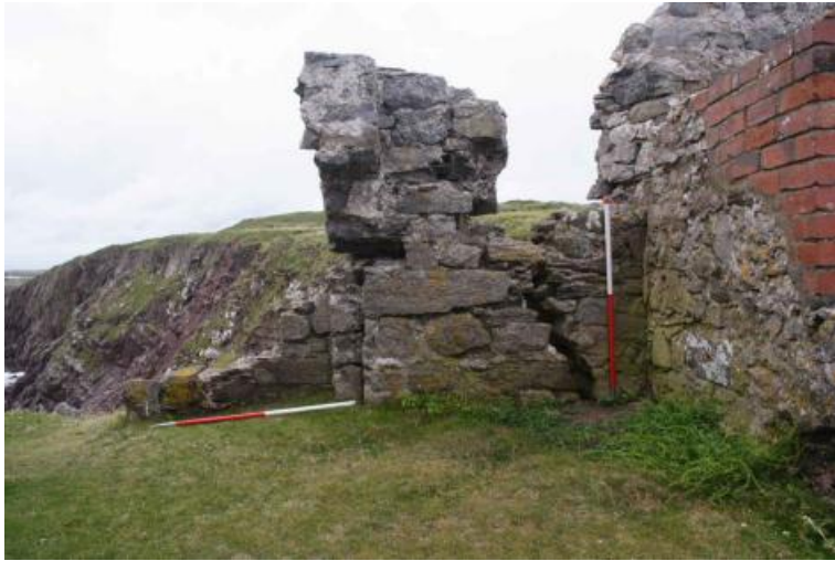
Photographs 13 – 15 General building recording photographs.
