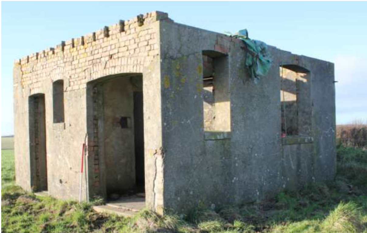
High Frequency Direction Finding station for Angle Airfield
