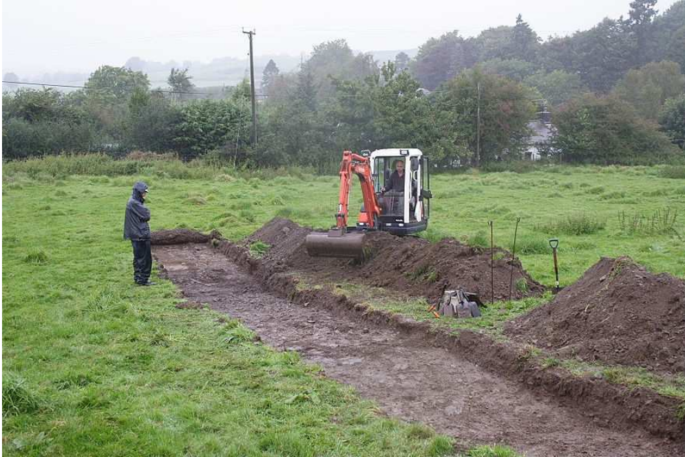
Photo 1: General shot of machine beginning to open the trench.
