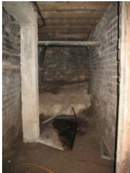
Concrete beam and column insertion adjacent to the south wall
