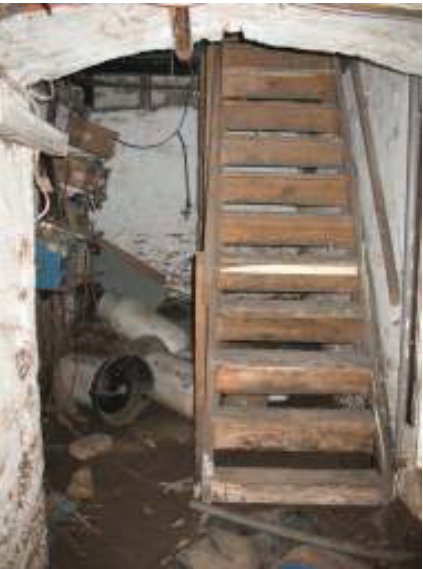
Room Bog – Timber Access Stair up to Ground Floor
