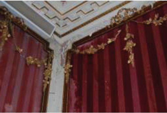
Red Drawing Room: Damage caused by water
