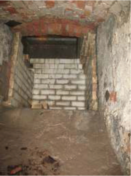
Light Well and Glazed Brickwork
