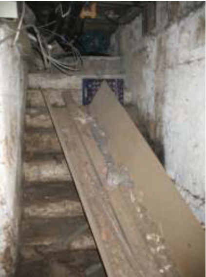
Redundant Solid Stair
